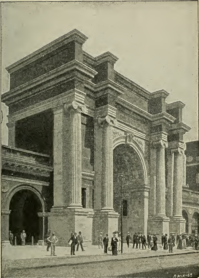
MAIN ENTRANCE, UNION STATION.
